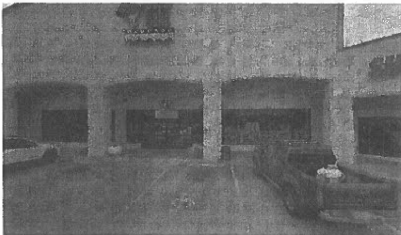
1009 S Jackson St Building
