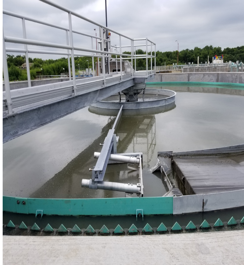
City of Ennis, TWDB WWTP Improvements
