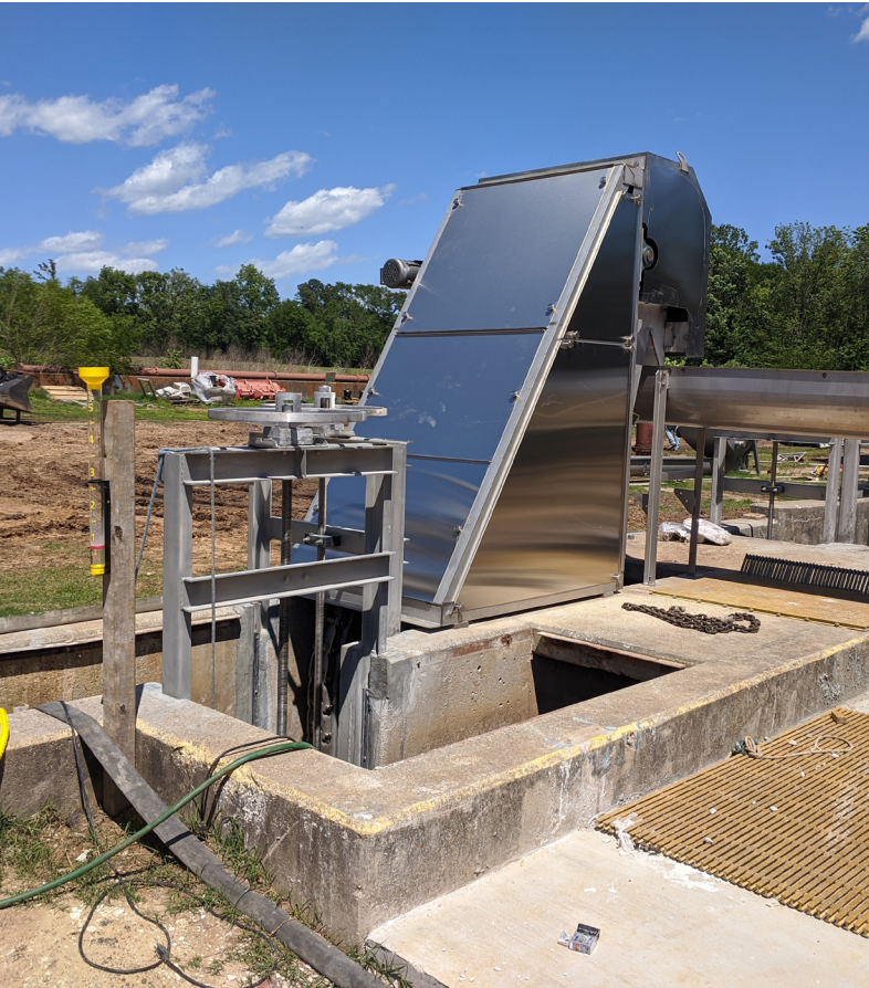
City of Gladewater, TWDB WWTF Improvements
