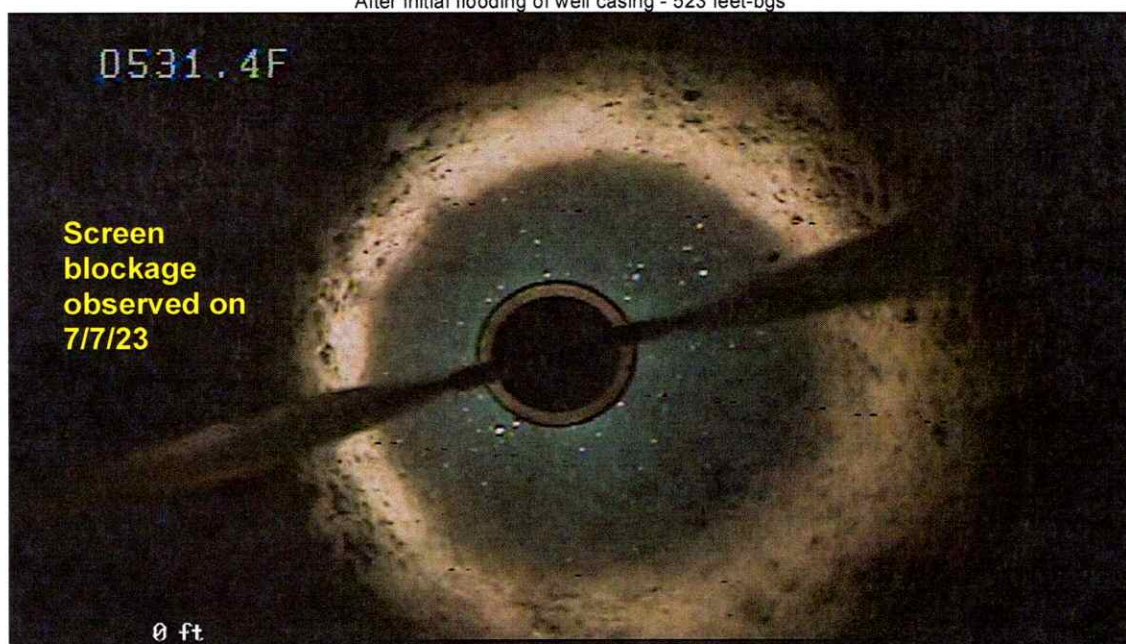
After additional flooding of casing - 531 feet-bgs
