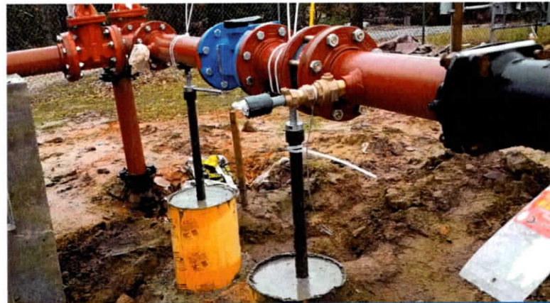
Kellyville-Berea WSC, Water Well Construction
