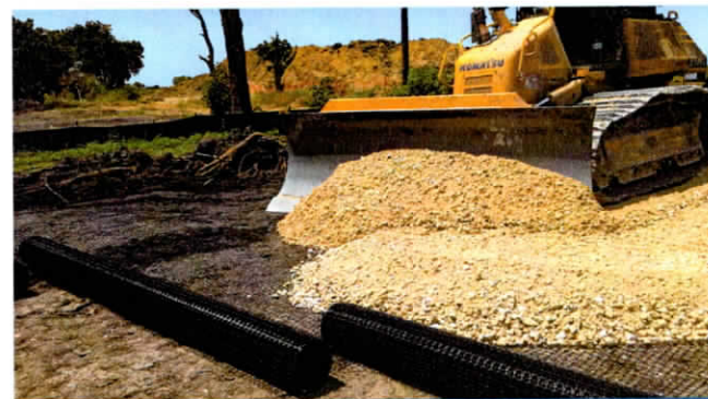
City of Alma, Sanitary Sewer Site Leveling
