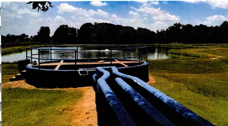
City of Alba, WWTF Improvements
