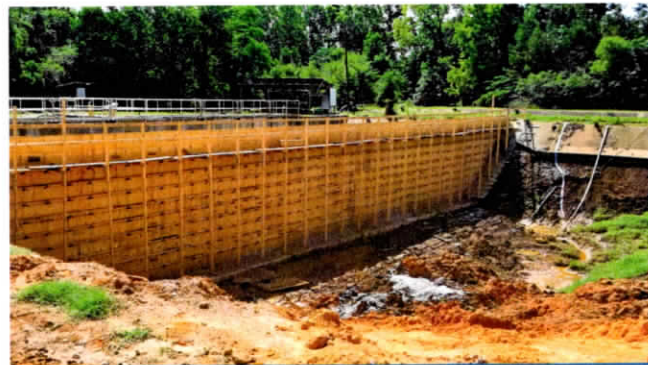
City of Alto, CDBG WWTP Improvements
