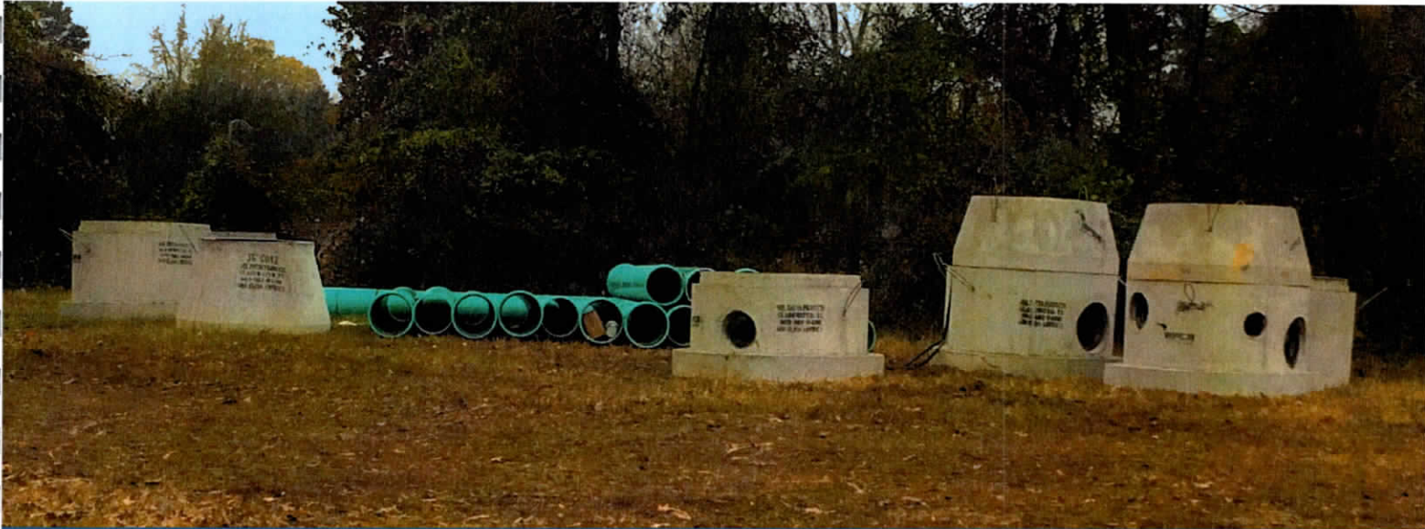
City of Jefferson, Sanitary Sewer Improvements
