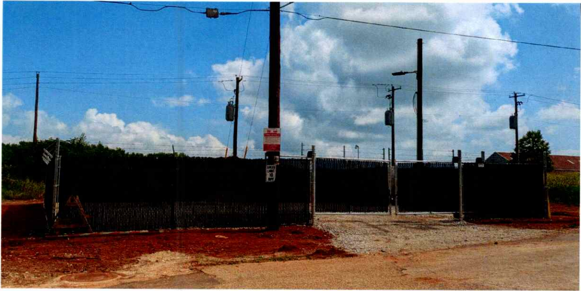
Sunnydale Lift Station – Exterior View
