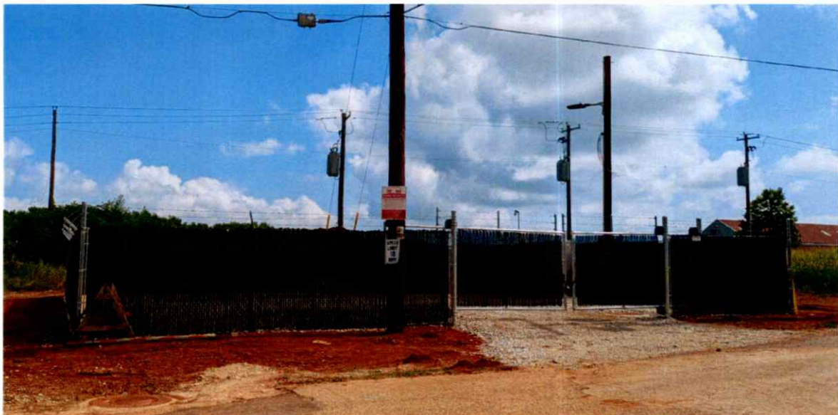
Sunnydale Lift Station – Exterior View
