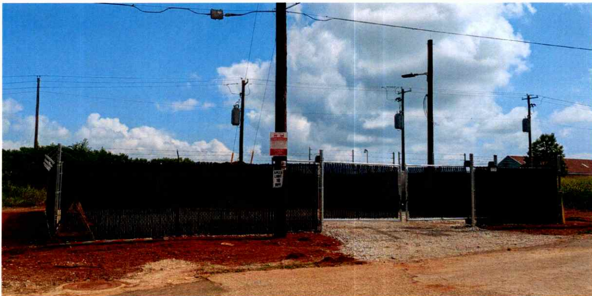
Sunnydale Lift Station – Exterior View
