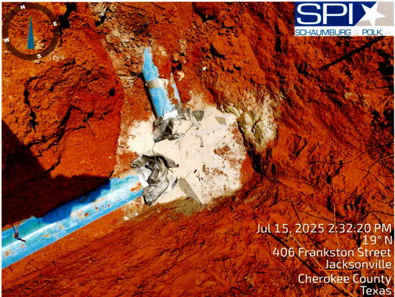
938042.00-250715- McKinney Moore putting in thrust blocks on the new water line.
